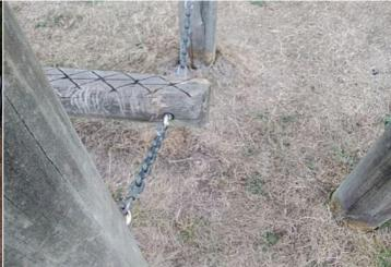
**Finding:** The ends of the beams do not have a minimum radius of 50mm as recommended in BS EN 1176 Part 1
