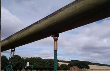
**Finding:** A number of fixing(s) have worked loose o the swinging steps
