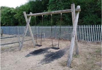
**Finding:** The inspector has some concerns about the internal condition of the timber crossbeam due to discolouration and was unable to verify the structural integrity without further testing. We recommend a Resi-PD survey to establish the condition of the timber at it's core.
