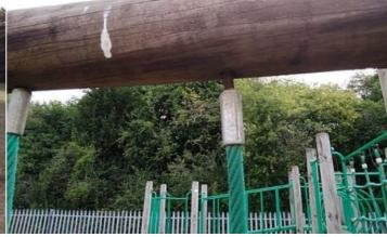
**Finding:** A number of fixing(s) have worked loose on he rope net
