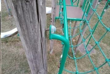
Finding: A number of fixing(s) have worked loose on the roe Action: Secure all loose fixings bridge
