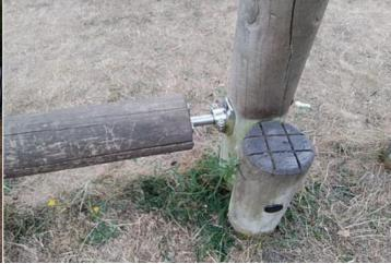
**Finding:** A number of fixing(s) have worked loose on the rotating beam brackets
