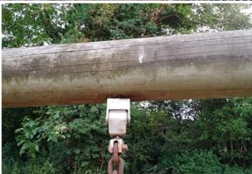
**Finding:** A number of suspension fixing(s) have worked loose
