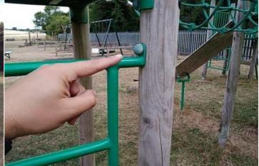
**Finding:** A number of fixing(s) have worked loose on the access element
