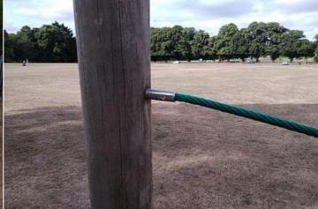
**Finding:** A number of fixing(s) have worked loose o the rotating beam rope grip
