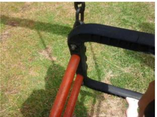
**Finding:** There are caps missing from the underside of **Action:** Replace missing caps under the seats the seats
