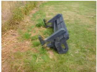
Finding: The bench is not securely fixed to the surface Action: and there is some possibility of the item tipping or rolling over
