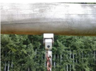
This design of swing joint has been known to fail on the weld connecting the joint to the Finding:
