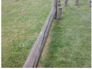
Finding: The timber on site has a number of splits (shakes) although these are not considered to be a problem at present
