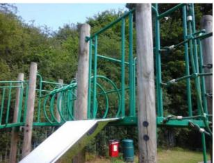
There is no side guard barrier to the slide start section and therefore does not conform to BS EN Standards Finding:
