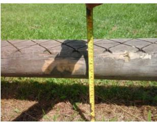
The clearance to the underside of the beam is **Action:** less than 400mm and fails the requirements of BS EN 1176 Part 1 Finding:
