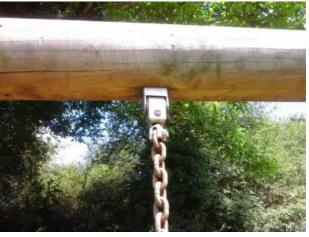
This design of swing joint has been known to fail on the weld connecting the joint to the threaded stud Finding:
