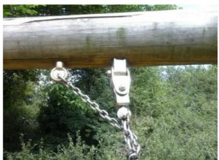
Finding: The suspension connection is loose Action: Tighten loose fixings to secure
