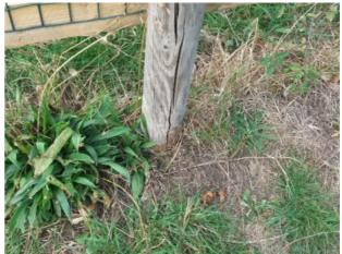
There is some strimmer / machinery damage apparent on the posts, this can penetrate the preservative applied to the timber and Finding:
