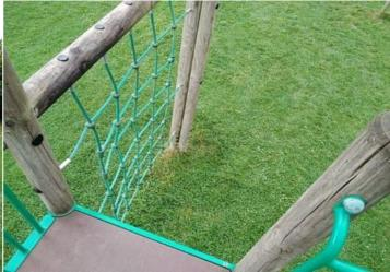
Finding: There is an opening in the barriers exceeding the Action: Monitor - No remedial work recommended width allowed (500mm) in BS EN 1176, and no guardrail has been provided; this is a low risk failure and no remedial action is required
