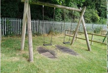
Finding: BS EN 1176 Part 2: Annex A makes a recommendation that fences or enclosures should be upto 1.50m from the edges of the swing seat to the sides, and subject to risk assessment, from the edge of the impact area. This is however, a low risk finding and no remedial
