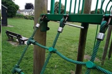
**Finding:** There is/are finger entrapment/s in the net and the **Action:** Monitor - No remedial work recommended item fails to meet the requirements of BS EN 1176 Part 1
