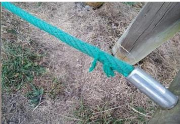
Finding: The ropes/nets are worn/damaged in places
