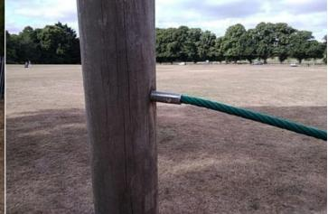
**Finding:** A number of fixing(s) have worked loose o the rotating beam rope grip
