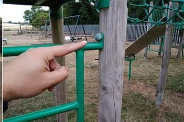
Finding: A number of fixing(s) have worked loose on the access element
