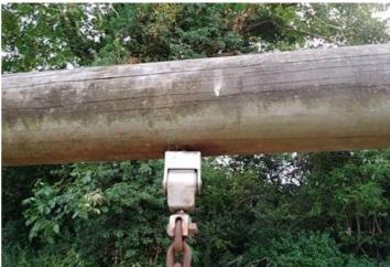
**Finding:** A number of suspension fixing(s) have worked loose
