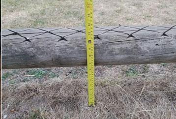
**Finding:** The clearance to the underside of the beam is less **Action:** Monitor - no remedial action recommended than 400mm and fails the requirements of BS EN 1176 Part
